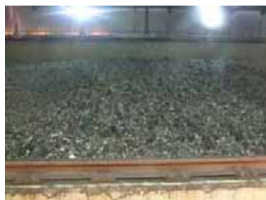
Mechanical Biological Treatment Facility
